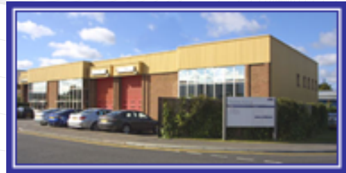
Kentec Training Center in UK (Dartford)
